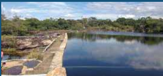
Wang E-Rang No.1 Dam
